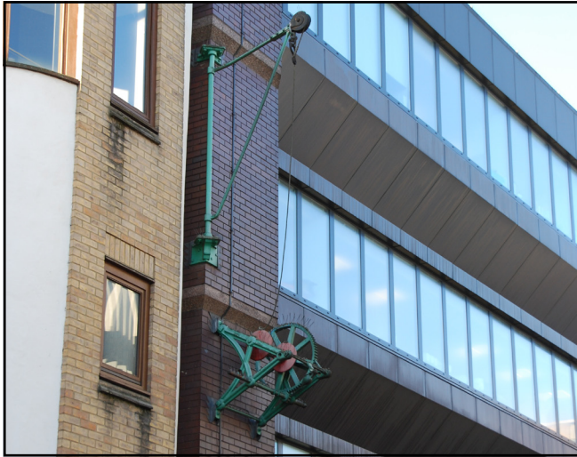
Figure 15: Former warehouse hoist on north-east elevation of CATs
